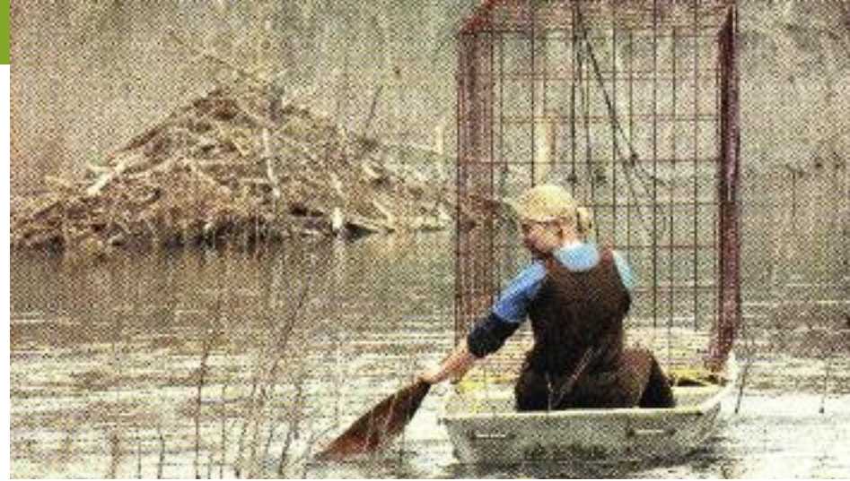
Beaver Impeders stop flooding caused by beavers. In this photo, a mesh protector—an essential part of the Beaver Impeder—is transported to the dam site by boat. (A beaver lodge is in the background.)
